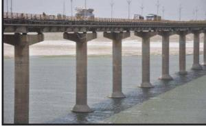
Constructed in 1976, the bridge has now aged close to 50 years. Even after undergoing several repairs, it is now deemed unfit for prolonged use. In 2021, a comprehensive repair project was undertaken, totaling approximately 4.62 crore rudiligent efforts invested to ensure its safety and longevity, the bridge deteriorated again within four months, leading to its closure in November 2022.
