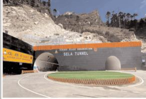
two main tunnels. The (T1) measures tunnels have been 1003.34m and the bored through the longer tube mountain at 13,116 1594.90m. Because of feet. They will reduce T2's length, the distance between 1584.38m-long Tawang and Dirang in narrower tunnel has been built parallel to it West Kameng district by to let users escape if 12km, saving almost 90 there's a cave-in.
